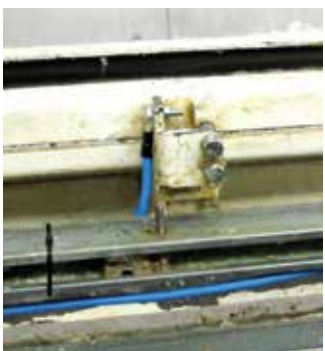
1 Connection of functional earthing system to painting booth
